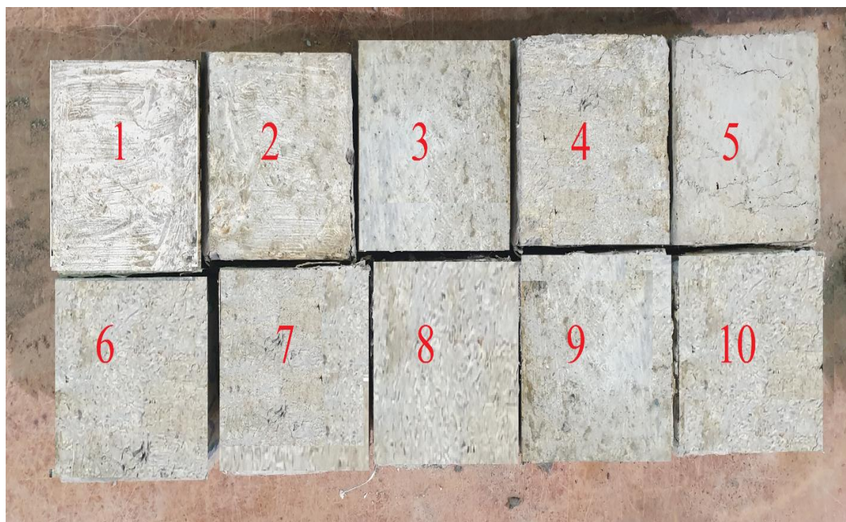
Figure 4. Visual inspection after the wetting-drying test
